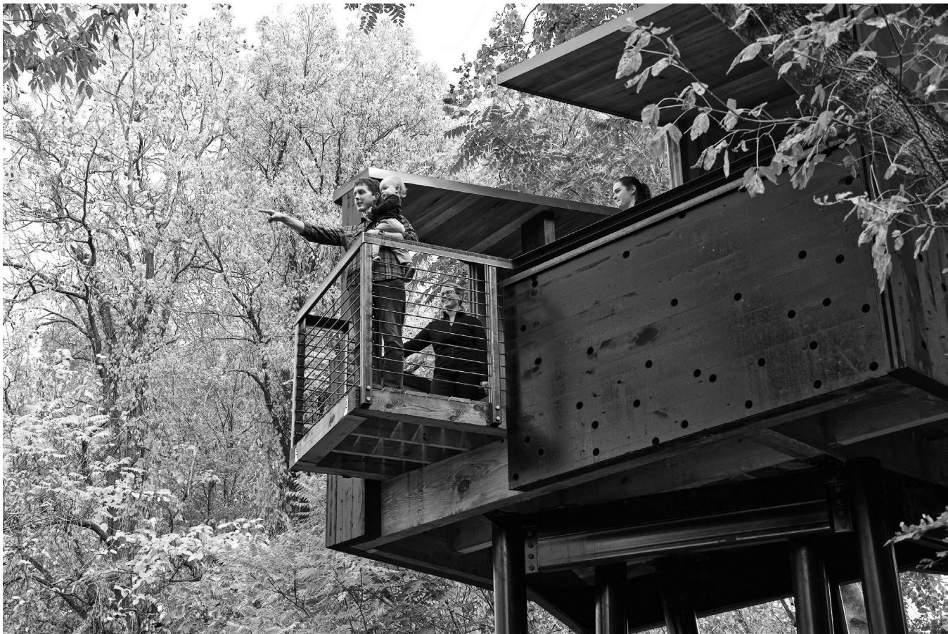
Figure 6: Radford Train Observation Tower, project co-led by author
