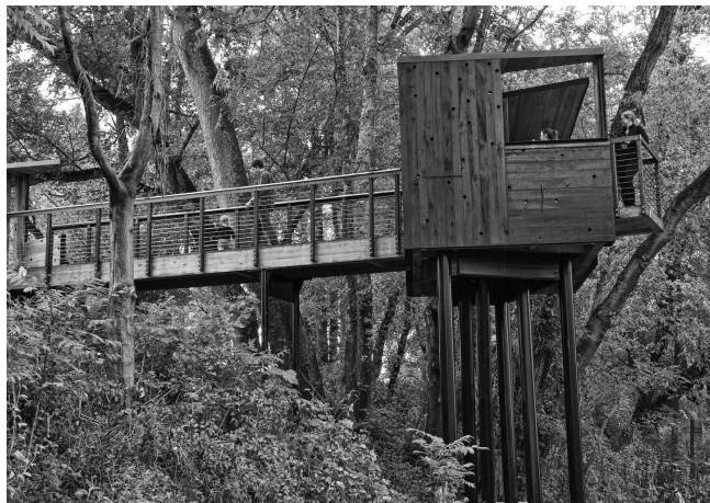
Figure 7: Radford Train Observation Tower, project co-led by author
